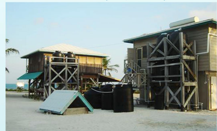
Rain Water System, Middle Caye
