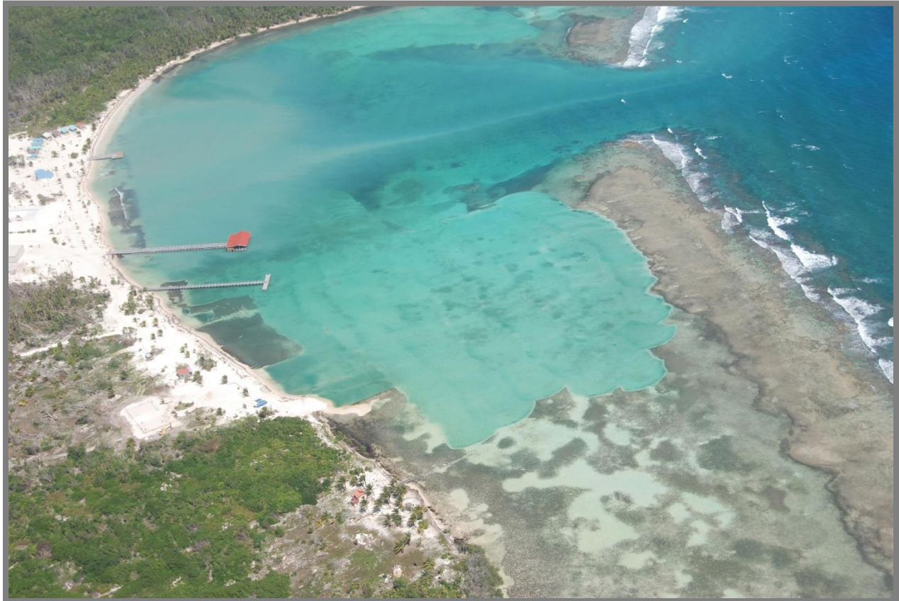
Figure 5: Dredging of Back Reef Flats at Ropewalk Caye
